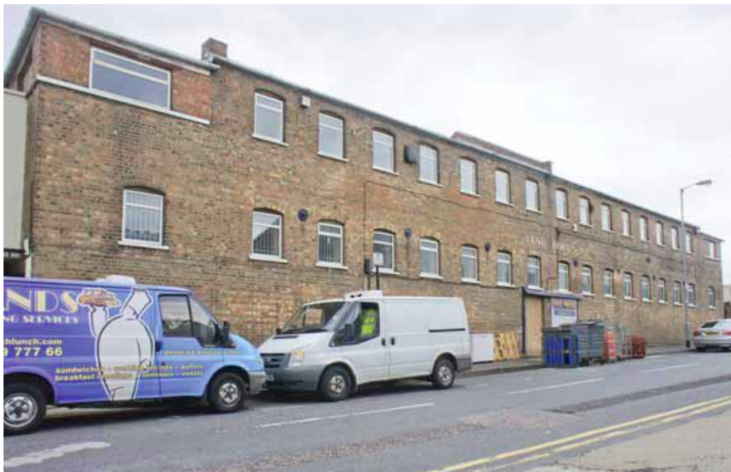
Tileyard Road (front) elevation
